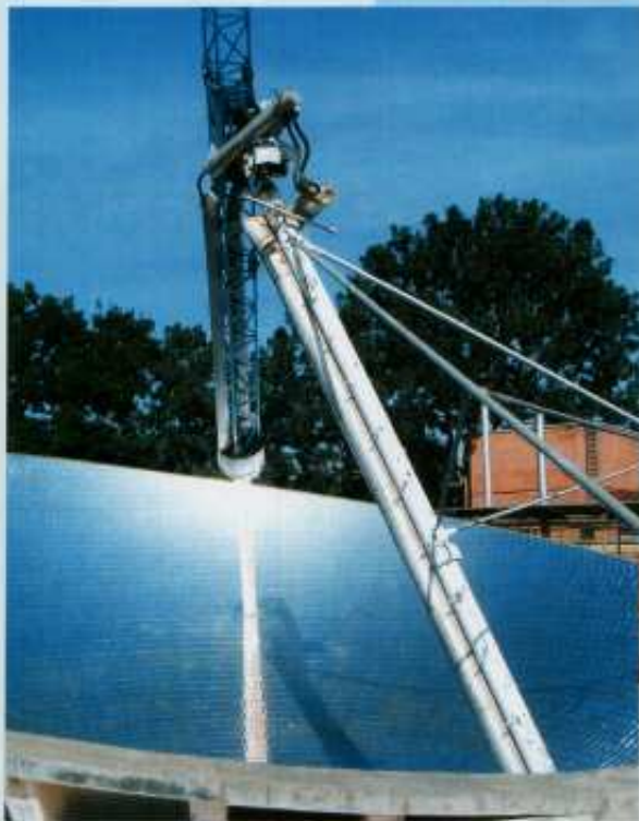
Water evaporator on the roof of the solar kitchen in Auroville
