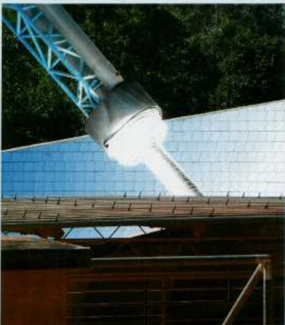
This collector produces steam for cooking in the solar kitchen. The receiver tracks the focal point of the sun.
