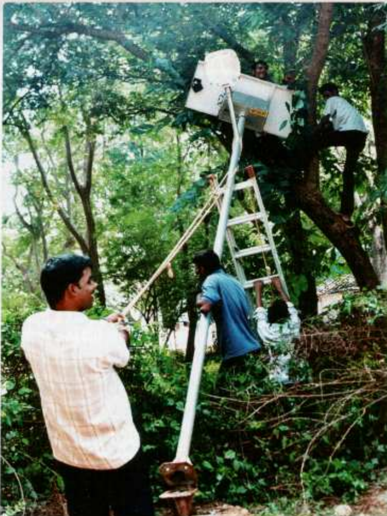
Workers setting up a solar streetlight
